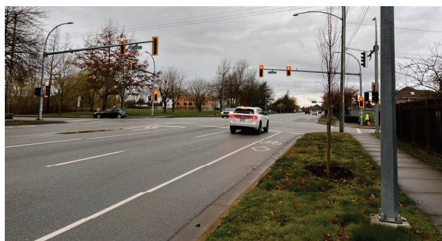
Westbound Ladner Trunk Road at 62 Street
