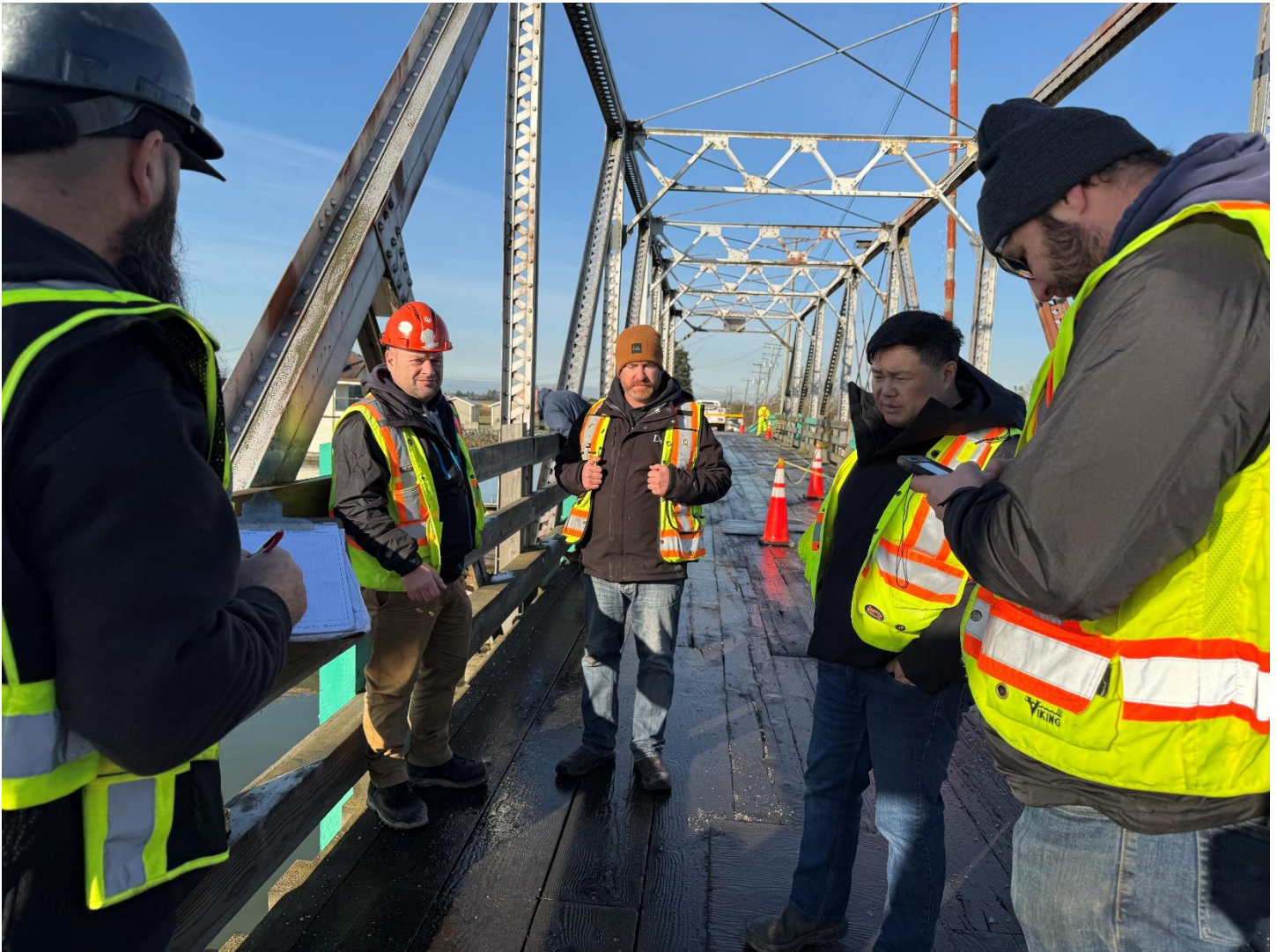
Photo 1: City of Delta staff convening, discussing watermain repairs needed
