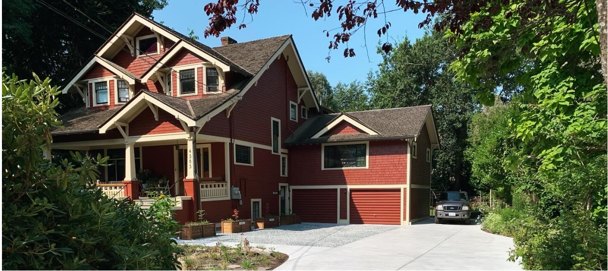
existing cedar roof
