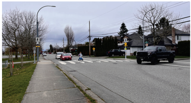
RRFB crossing at 62 Street and Holly Park Drive
